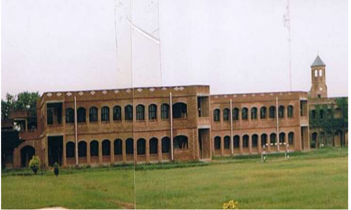
Chand Bagh School Sheikhupura Road, Muridka.
